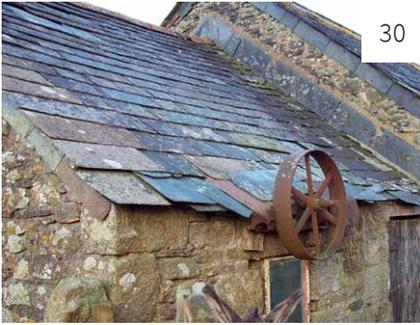
**Image 30: Slate** for roofing could traditionally be obtained only from parts of Wales, the Lake District, the West Country, Leicestershire, and the Isle of Man. From the late-18th century onwards Lake District and Welsh slate was carried far and wide as a result of improved canal, coastal shipping and rail networks. Slate was also used to clad the walls of some farm buildings, most notably in Cornwall, West Devon, and Cumbria.
