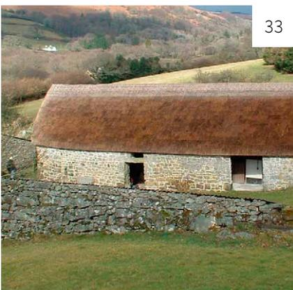
**Image 33: Thatch** was historically the most widespread material for roofing farm buildings, although its method of application varied from region to region and according to the available raw material. Long straw and combed wheat reed (also called Devon reed) were the most common, but heather and water reed were also used in areas where they grew naturally.
