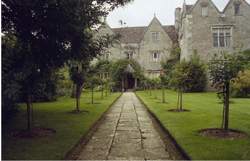
Kelmscott Manor, Oxfordshire (Grade II)
