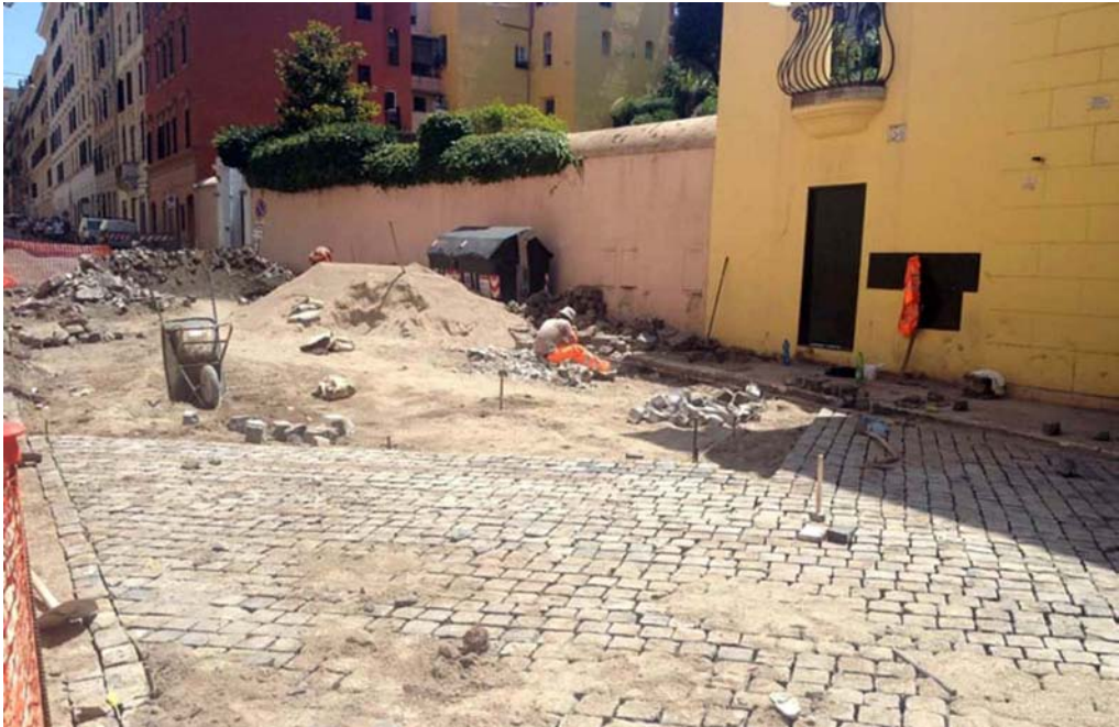
Figure 5. A street being re-setted in Rome, Italy. Photo: author
