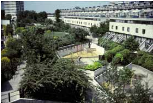
The re-furbished Alexandra Road Park, c 1980
