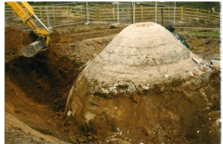
2 The Ice-House Dome at the start of excavation, looking west
