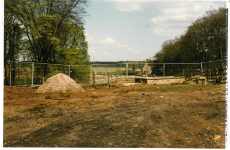
The Ice-House Dome looking east
