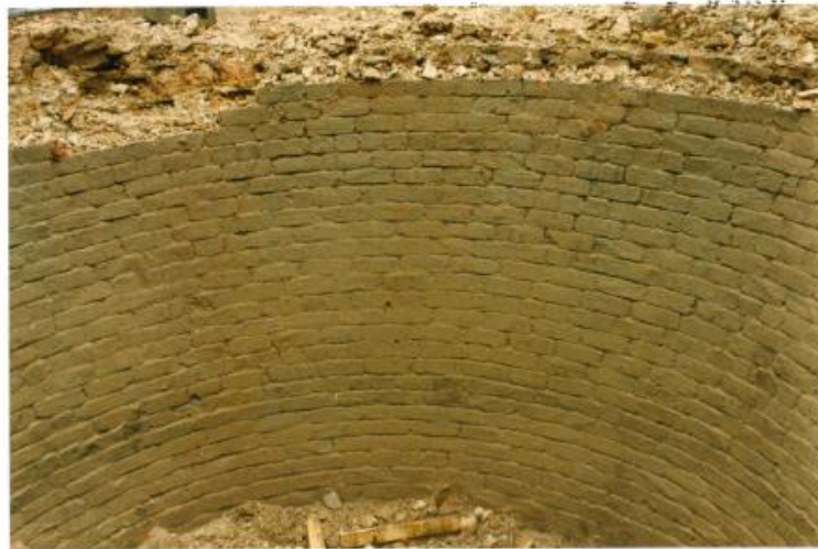
17 Detail of interior brickwork at base of ice-house structure.
