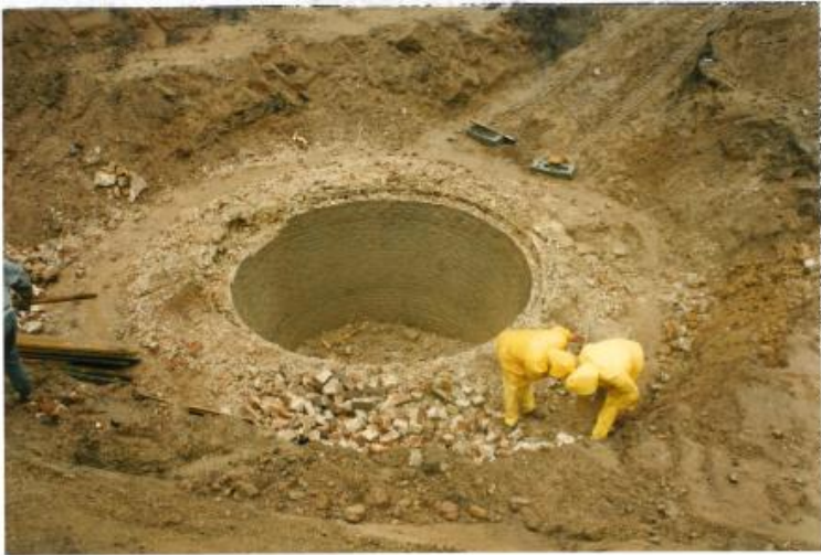
16 Final excavated depth
