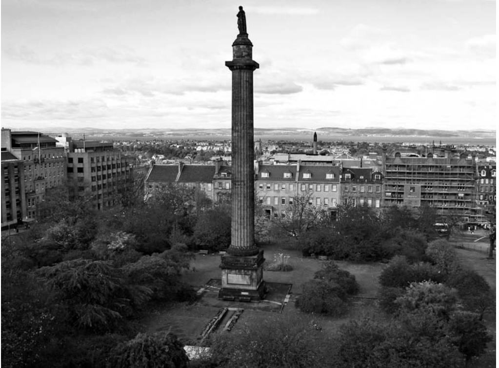
Figure 1. St Andrew Square before work began – clearly showing the avenue of ornamental trees introduced in the post-war years. Courtesy: Reproduced by permission of City of Edinburgh Council, late twentieth century
