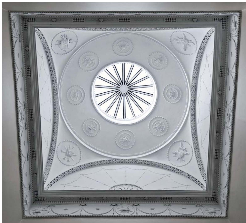
Figure 6. James Nisbet, George Street, cupola. Photo: Carsten Flieger, 2011. Lady Balcarras instructed Nesbit to decorate her New Town houses in 'an elegant and handsome manner, such at least as is usual for houses in the New Town of Edinburgh to be built'. The stucco was to be 'uncommonly elegant'. Nisbet gave it the same moulds as those he gave the Queen Street houses he built with builders such as Robert Inglis and other members of the Society of Master Builders of Edinburgh
