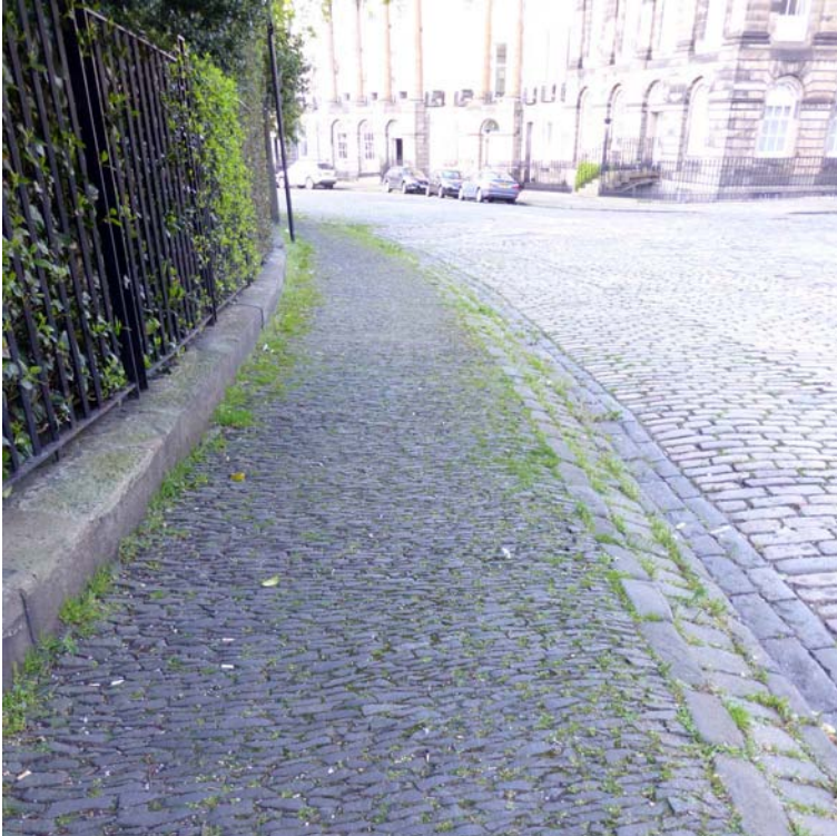
Figure 7. Moray Place – an incredibly rare and precious survival, the ‘horrorized’ path of c.1820 that completely encircles the circular garden of Lord Moray’s Pleasure Ground
